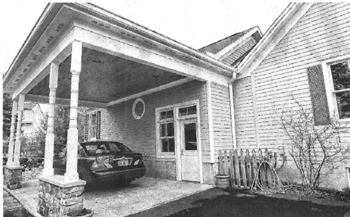
DeVol added a carport that protects his father-in-law from inclement weather when coming and going from his new, aging-in-place apartment.
